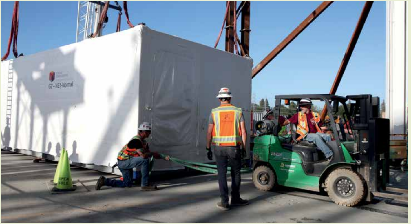
Prefabricated modular units arrive at Bay View and are readied for stacking as part of the short-term corporate accommodations.
