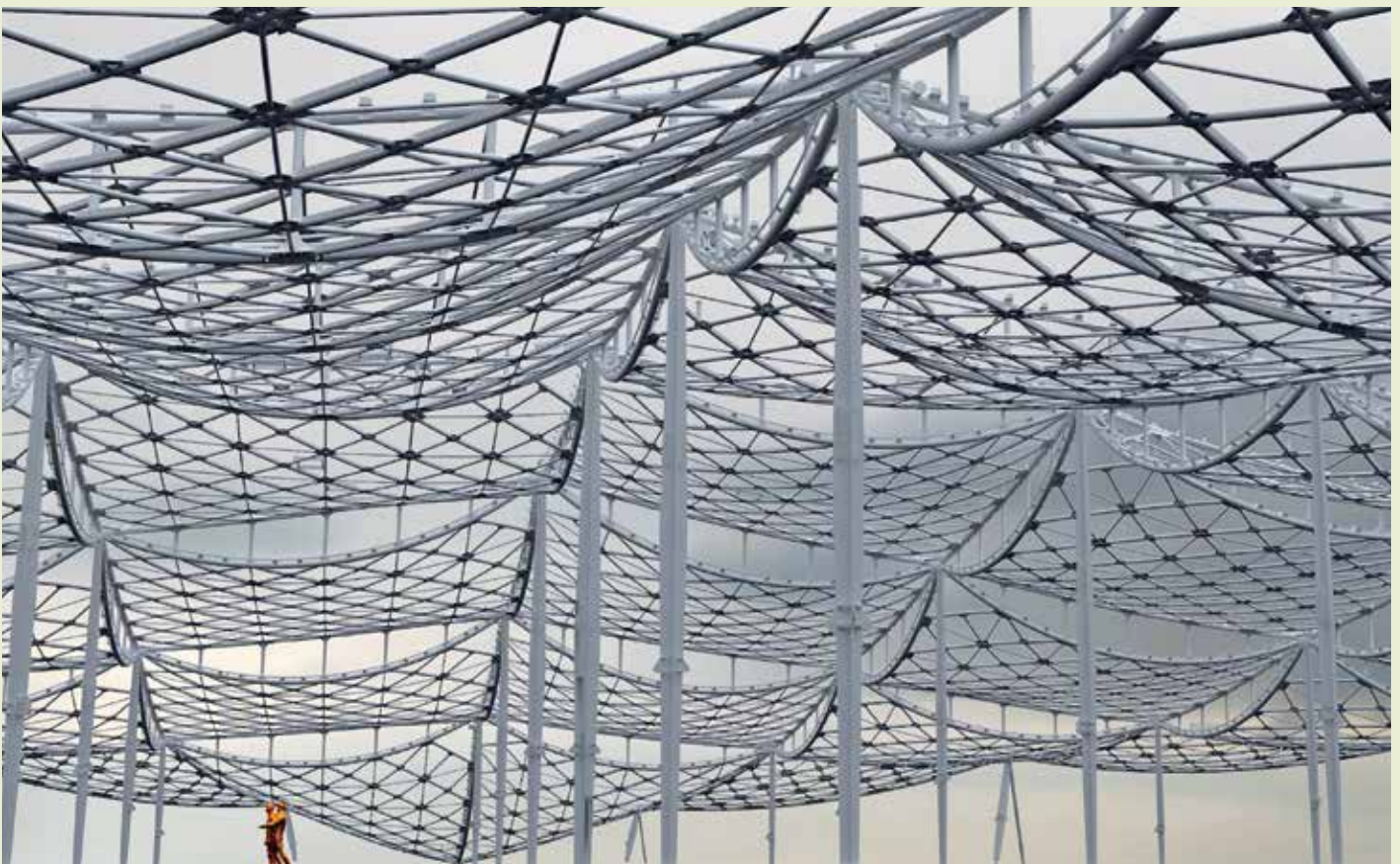
A structural model of the canopy showing the tensile bays and clerestory trusses spanning between a field of slender columns.
