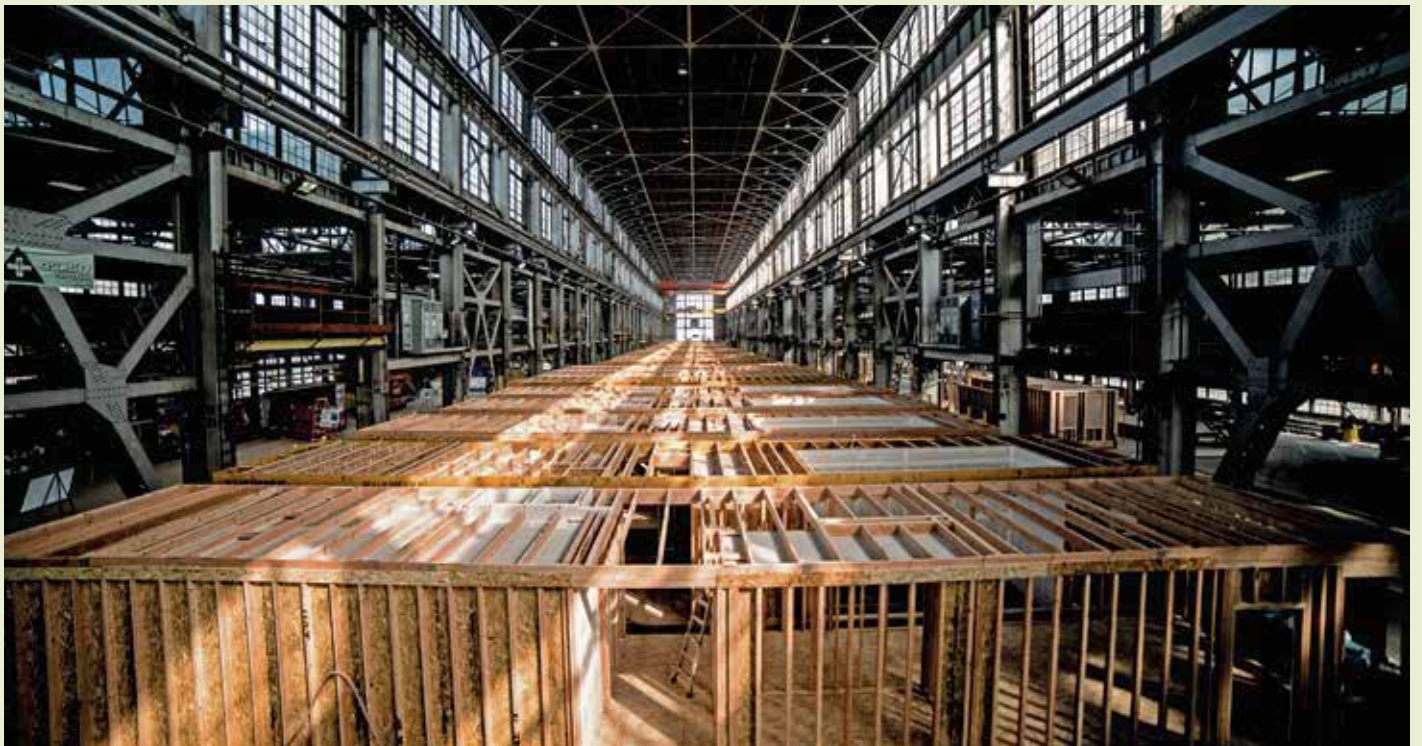
An interior view of the Factory_OS operation in Vallejo, California, where the company produces prefabricated modular housing units at scale.
