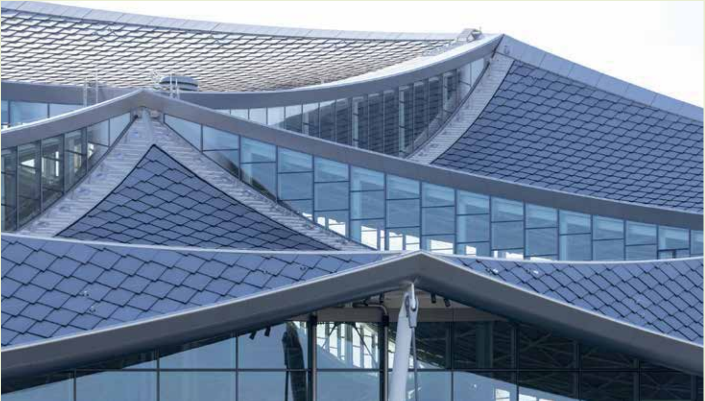
A close-up of the dragonscale building integrated photovoltaic system that aims to make solar part of the architecture rather than an add-on.
