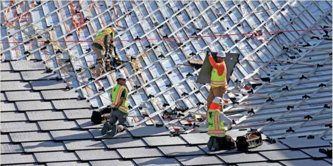
Contractors continue the installation of the dragonscale solar skin.
