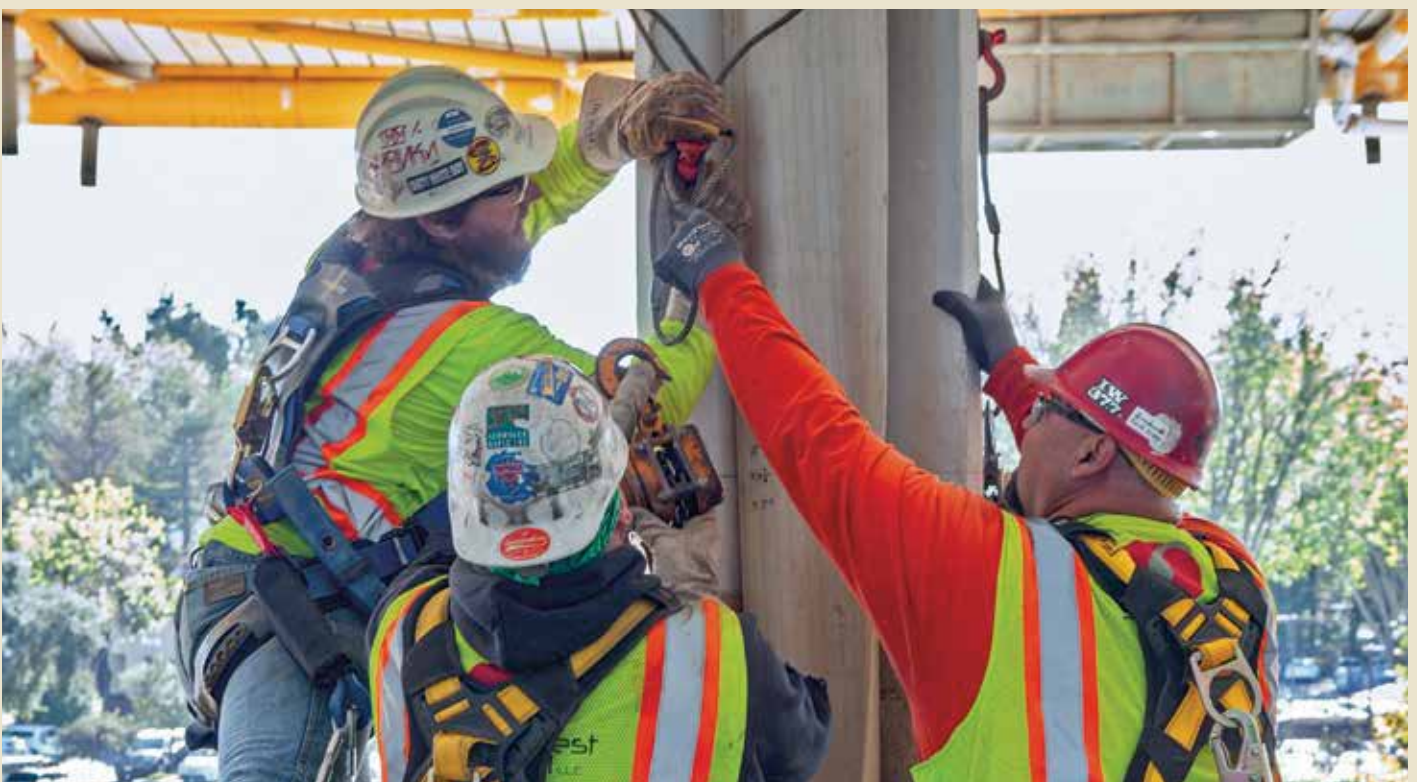
A team of contractors problem solve at Charleston East.
