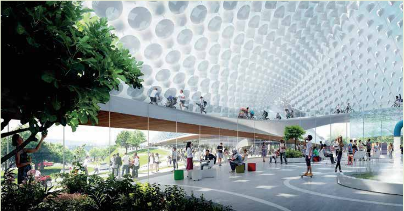
An early rendering showing the concept for a structural ring beam that supported the canopy while providing a circulation loop for bikes and pedestrians throughout the building.
