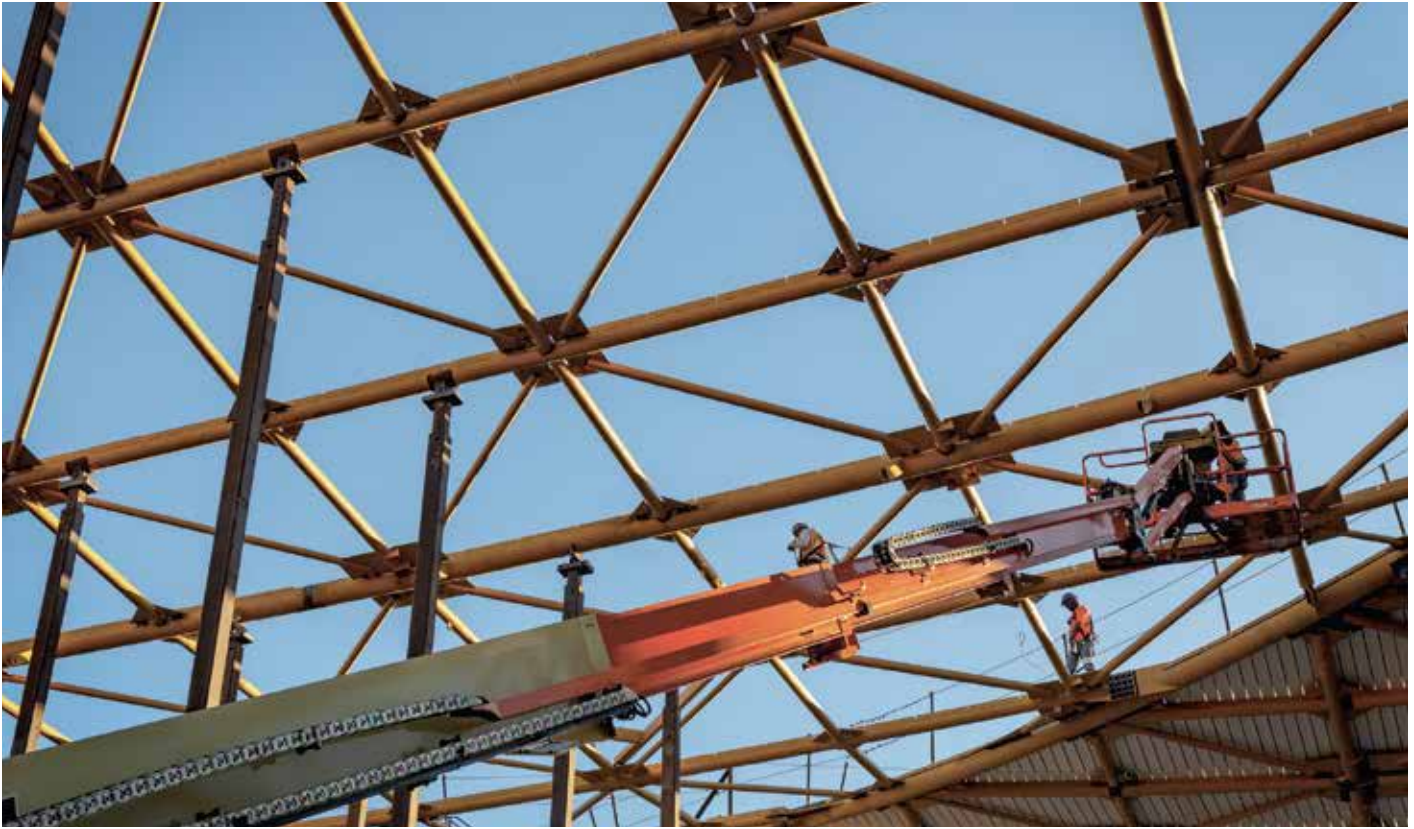
Above: “Tube net” steel is in place as work on the roof is advanced at Charleston East.
