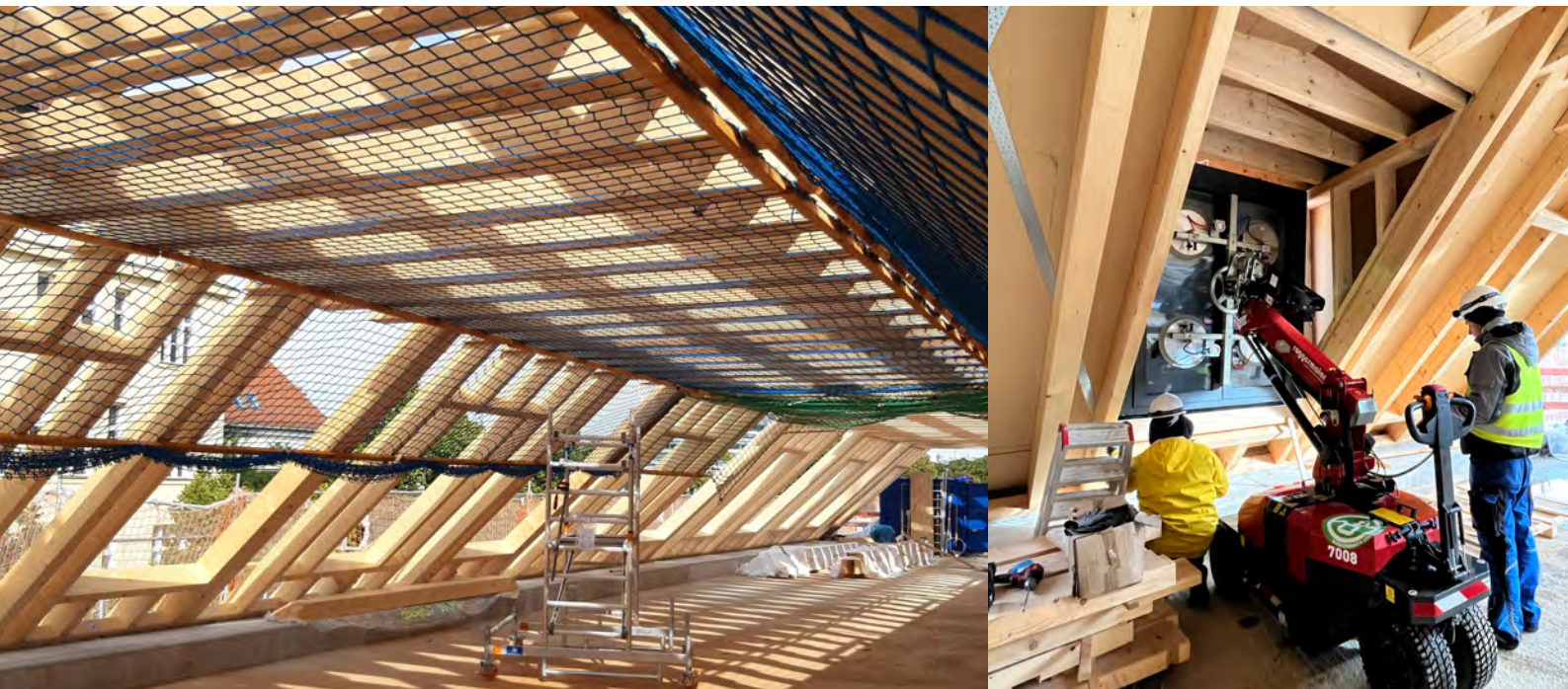
Wing building's new wooden roof at initial structure stages
